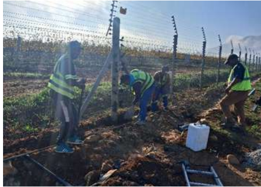
The Estate's Security Department initiated the next phase of the fence upgrade project. PHOTO: Supplied.
