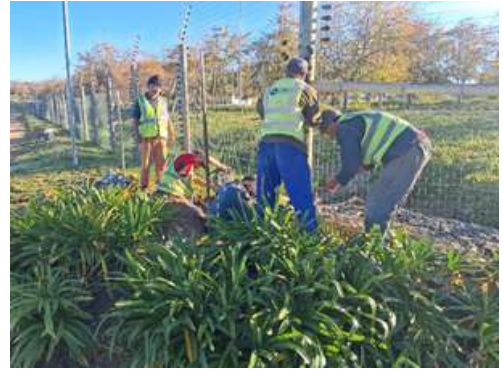
BSM Projects replaced fence posts, stays, and strands in selected perimeter sections. PHOTO: Supplied.
