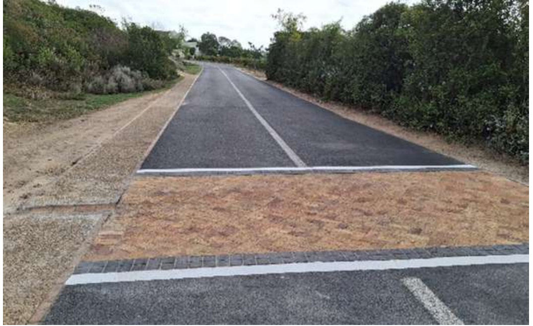
A new speed bump was installed leading to De Vleie to help reduce speeding violations within the village. PHOTO: Supplied.
