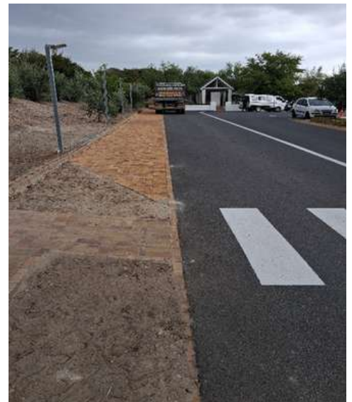
An additional lane was added to the Contractor's Gate to prevent traffic congestion at the Estate's main entrance. PHOTO: Supplied.
